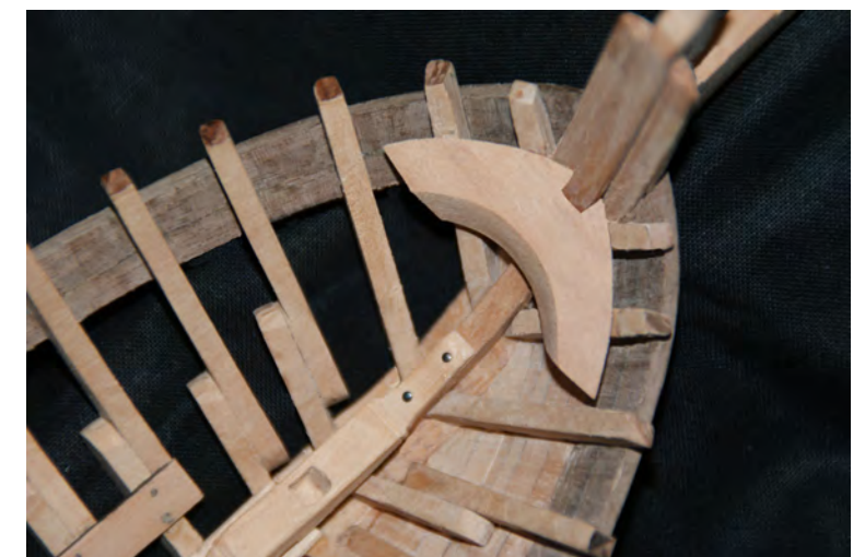
Photo n°. 34: Installation of the breast-hook (25). The notches for the deck clamp (one on each side) are still to be cut. Note the foremast step on top of the keelson, above the keel.
